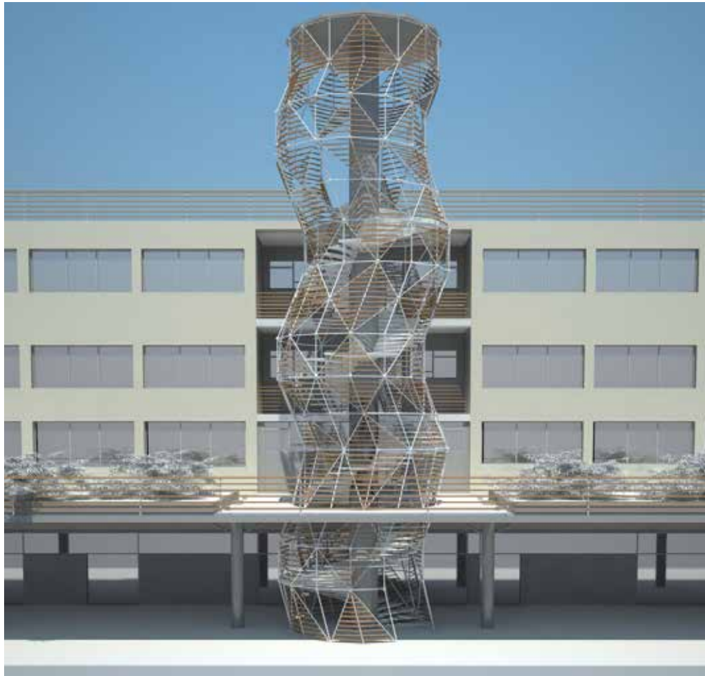
One of the main elements of the reuse project is the renovation of the emergency staircase, positioned at the center of the building, toward the train tracks. The new spiral staircase is supported by a lattice structure that allows it to grow through through a particular form inspired by the "tower of the restaurants" Ridolfi.
