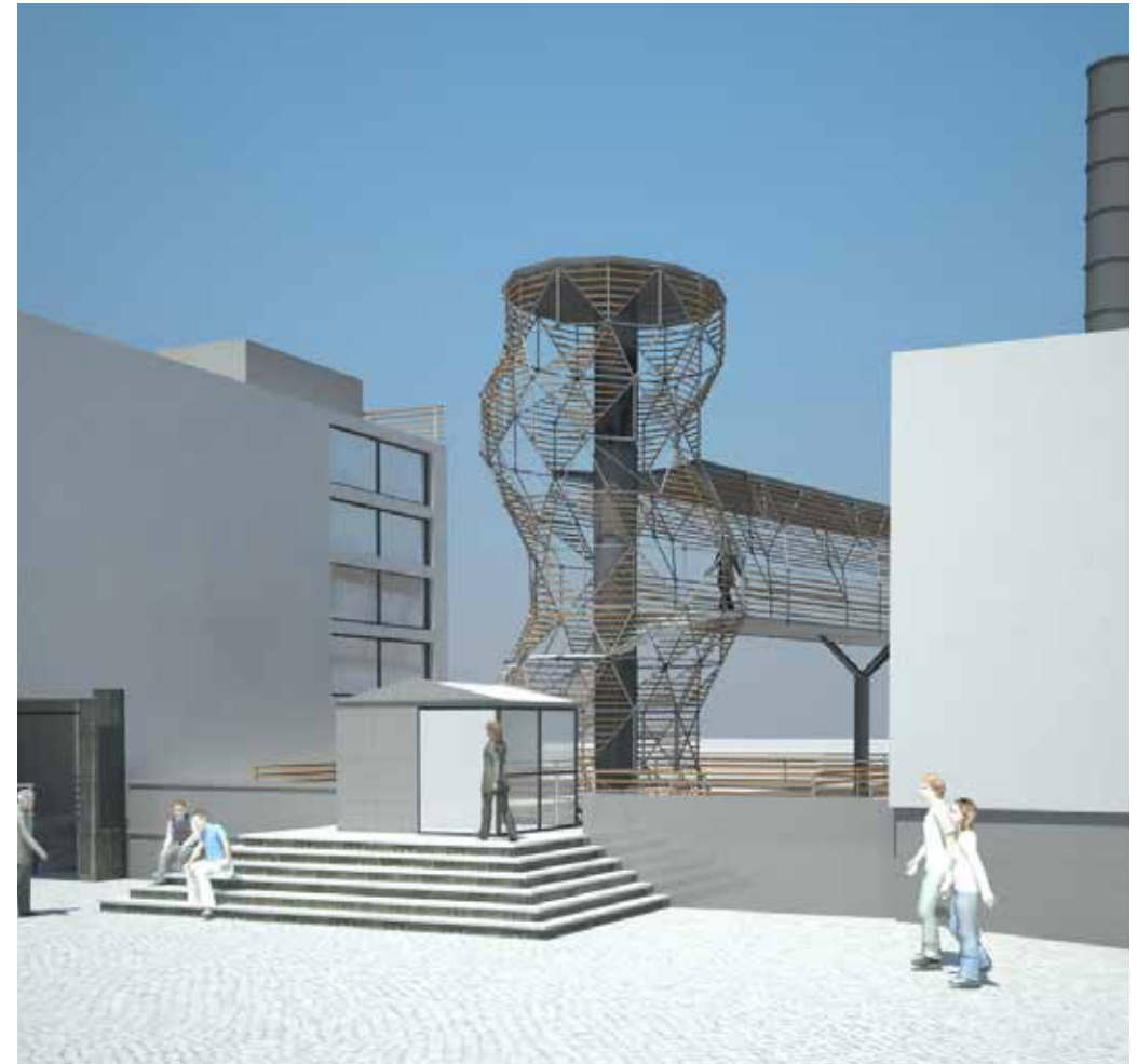
In addition to the emergency staircase, the project includes the construction of 4 more stairs that connect the rails' level to the road (in this case: Via Ferrari). Through these stairs is also possible to reach a bridge that crosses the train tracks, connecting Via Ferrari to the Isola district.
